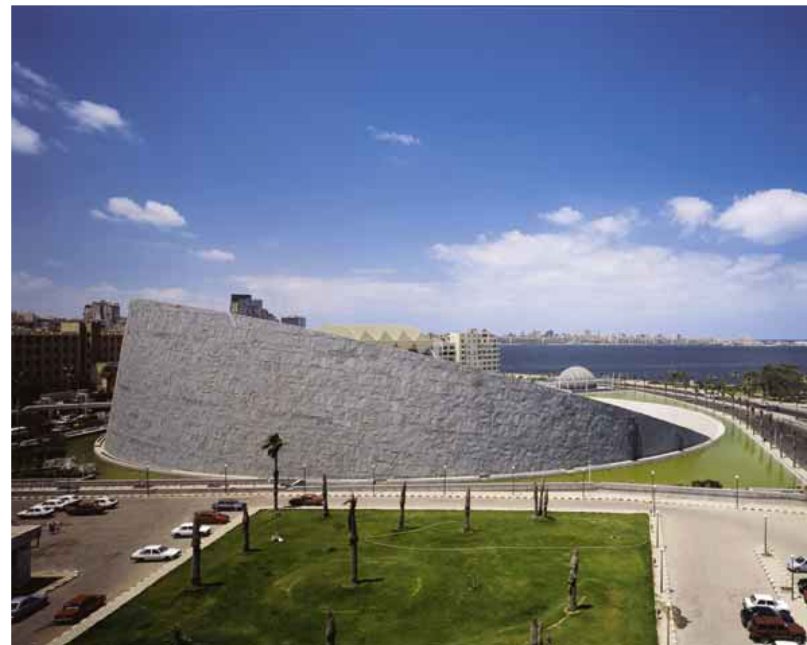
Specially made aluminium screens, left, shield the library from the direct effects of the hot Egyptian sun. Partly sunk into the ground, the distinctive elliptical shape of the library's drum is the culmination of Alexandria's sweeping coastal road, above
